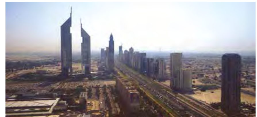
Potemkinkorridoren Sheikh Zayed Road med The Twins »Emirates Towers«
