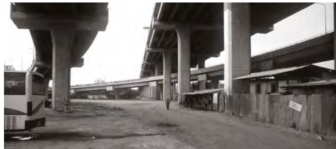
Outlanders under Inthra Expressway
