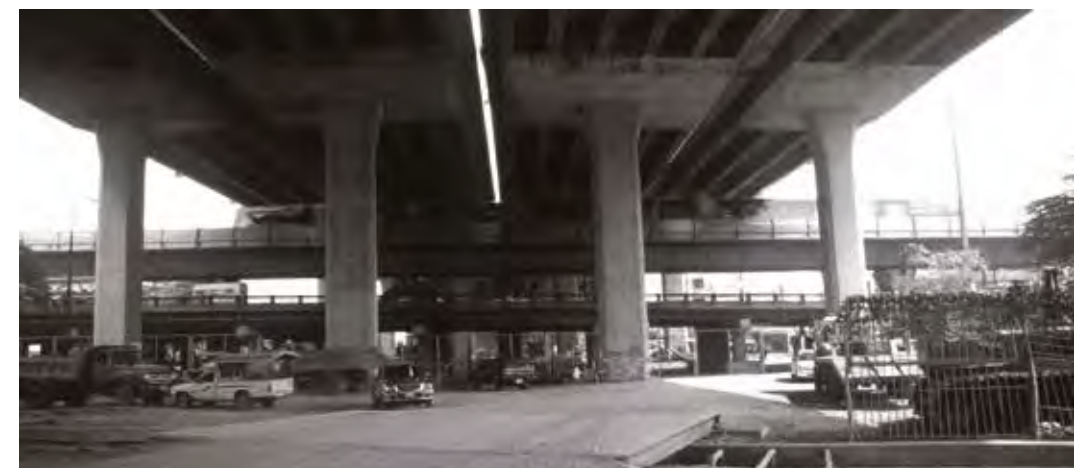
BTS krydser under Inthra Expressway
