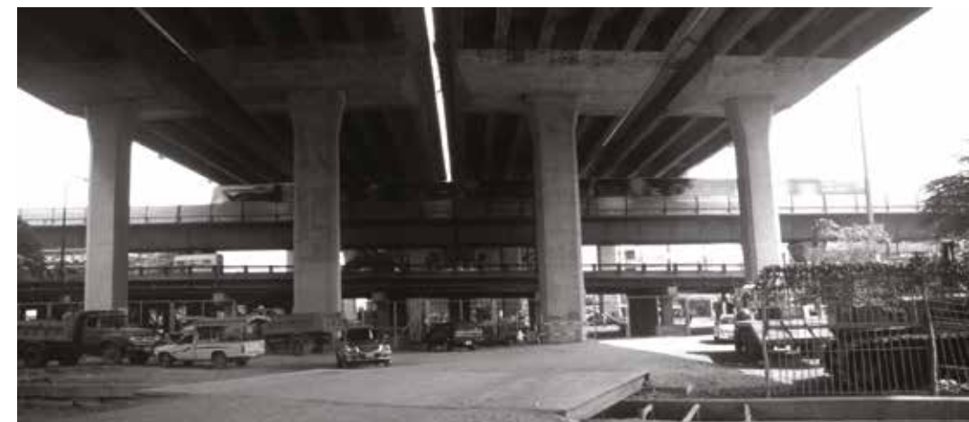
BTS krydser under Inthra Expressway
