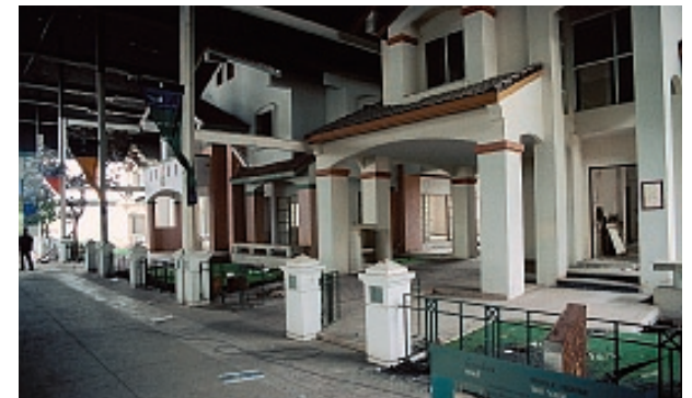
Inside the cracked "Expodome Home Center", Bangkok.
