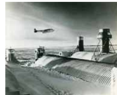
Camp Century was a nuclear powered research center built by the US Army Corps of Engineers. The camp was evacuated in 1966. Movements in the ice sheet made the trenches difficult to maintain.
