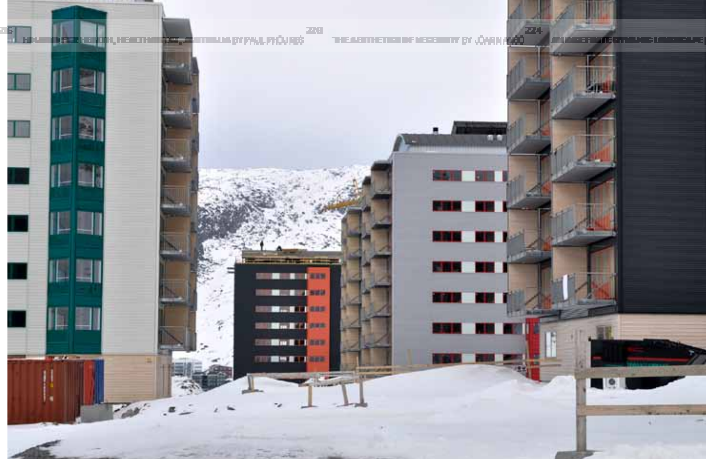
The subject of the plan 4A5-2 under construction. The perfect spot for a tranquil stone garden one might think.
