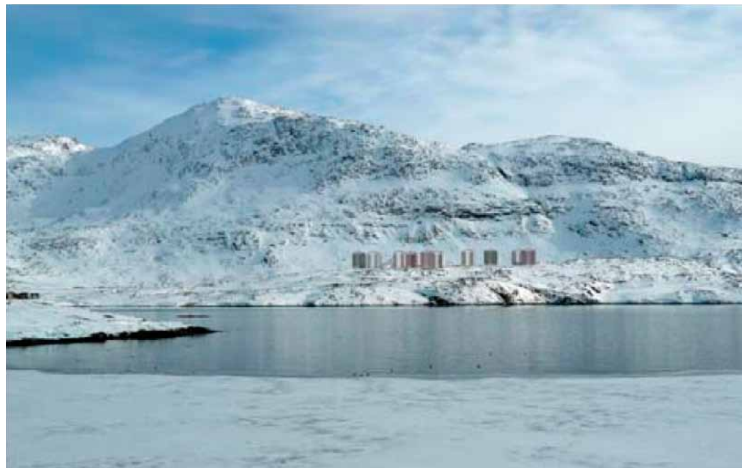
The structure pasted on a snowwhite landscape seen at a distance of 2 km.
