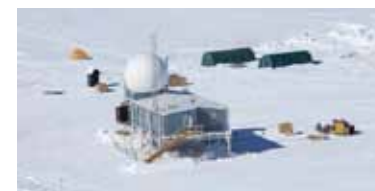
"Big House" at Summit Station is the main building in the station and houses dining and recreational areas for the staff as well as kitchen and offices.
