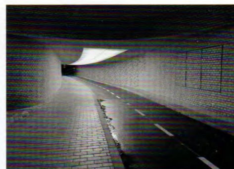
Ny tunnel under Nørrebrogade. AART Architects. Foto: Boris Brorman Jensen
